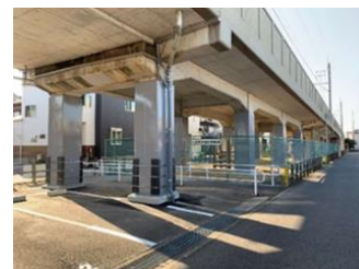
Seismic reinforcement for elevated bridges
