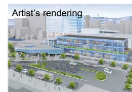
South gate (completion slated for FY2023)
